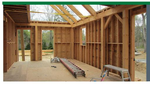
Above-grade walls consist of doublewall construction with two 2x4 16-inch on-center framed walls set next to each other to provide a 7-inch-thick wall cavity for R-25 of blown-in fiberglass insulation. The stud walls are staggered to prevent thermal bridging through the wall. A coated OSB sheathing product provides air sealing and a drainage plane behind the clapboard and cedar shingle walls.
