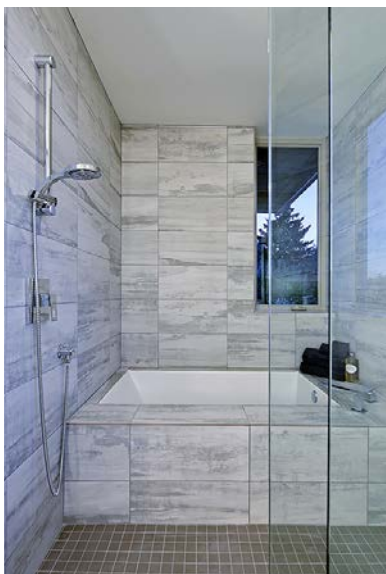
All of the home's plumbing fixtures are EPA WaterSense-labeled.
