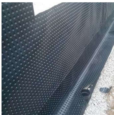
Plastic drain mat protects basement walls from water infiltration.
