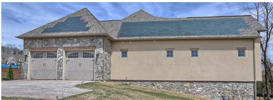
Solar PV shingles integrate seamlessly with the roofing shingles.
