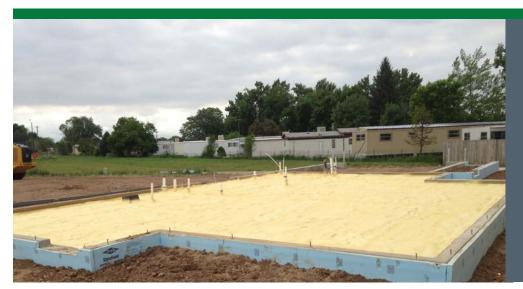
For enhanced comfort and reduced energy, the townhomes' foundation is wrapped in insulation. A thick R-60 layer of spray foam blankets the ground under the slab while slab edges are covered with an R-10 layer of rigid foam.
