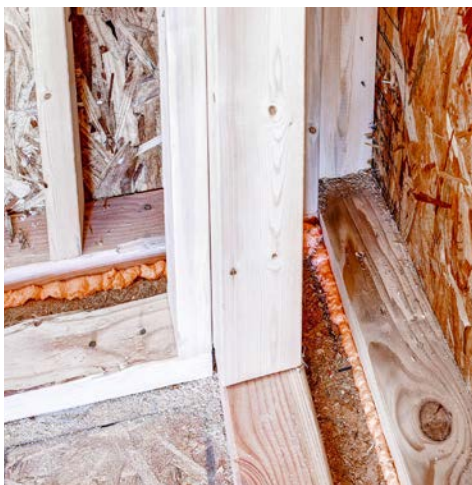
The double-stud walls will hold 9.5 inches (R-40) of blown fiberglass.
