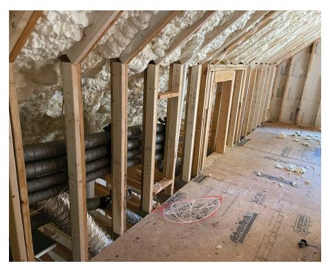
The attic is insulated on the underside of the roof deck with 8 inches of open-cell spray foam, providing an insulated space for the small-diameter HVAC ducts as well as additional living space.
