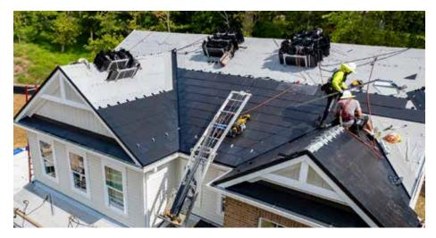
The entire roof of the home is covered with photovoltaic panels. The panels provide 10 kW of solar power and, together with the 27 kWh of battery storage capacity, enable the energy-efficient home to yield near net-zero energy bills over the course of the year.
