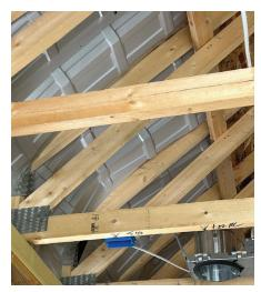
Baffles and wind dams provide a path for airflow from soffit vents to ridge vents, cooling the underside of the roof to reduce the risk of ice dams in winter.
